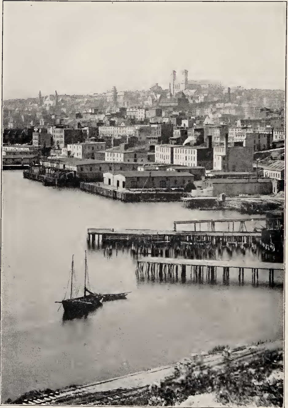
St. John's, the capital city of Newfoundland, sits high on a hill overlooking the land-locked harbour. It is the centre of the fishing industry, and the commercial metropolis of the island. Its atmosphere is distinctly British.
